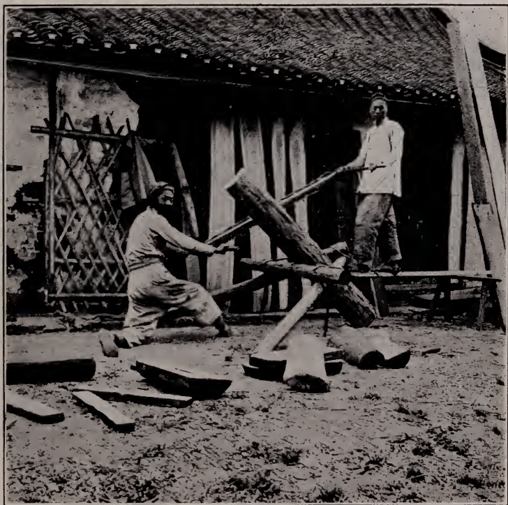
FIG. 28. — Usual method of sawing lumber in China.
