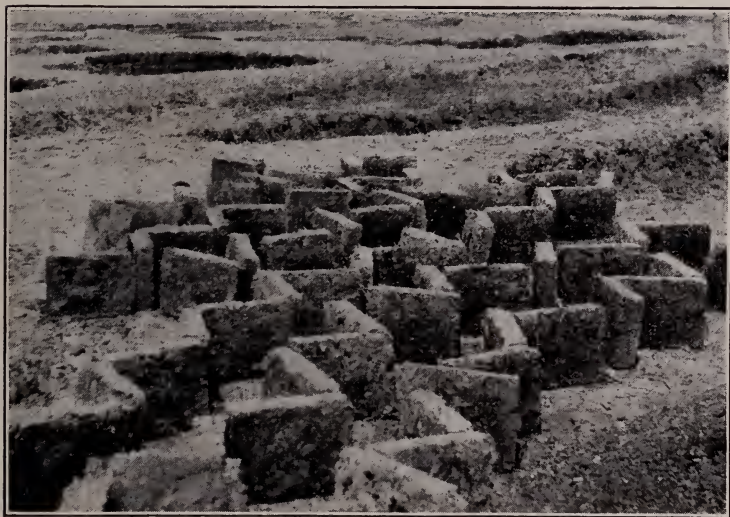
FIG. 74. — Air-dried earth brick for house building.
