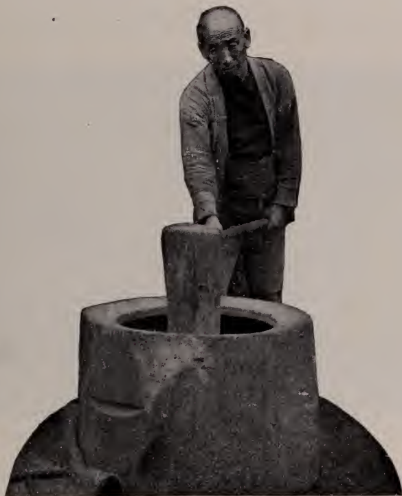
FIG. 160. — Large wooden mortar used for the polishing of rice in Japan.
