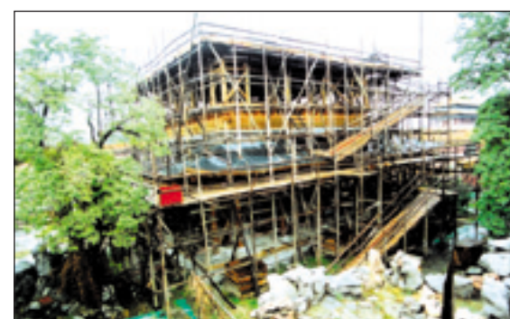
Yanchun Pavilion under construction
