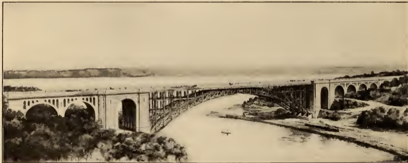
HENDRICK HUDSON MEMORIAL BRIDGE, to be erected over Harlem Ship Canal (Spuyten Duyvil), by the City of New York, to commemorate in 1909 the Ter-Centenary of the discovery of the Hudson. Designed by Alfred P. Boller; length, 2,500 ft.; central span 820 ft.; clear height, 175 ft.; estimated cost $5,000,000. Connects Riverside Drive Extension with Spuyten Duyvil in the Bronx.
